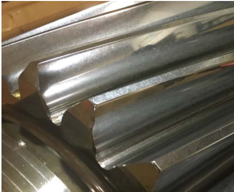
Fig. 43 Close-up of ISF repaired intermediate pinion
