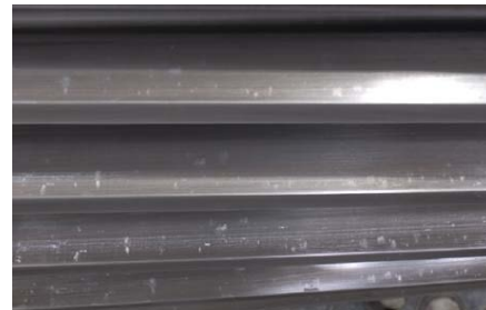
Fig. 17 Example of FOD Damage on a Wind Turbine Annulus Gear
